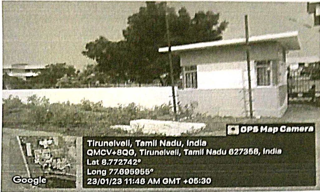
7.1.2 (a) 5.College Compound Wall
