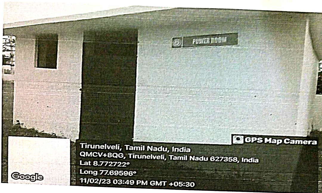
7.1.2 (a) 10..Generator for Power back up and Server
