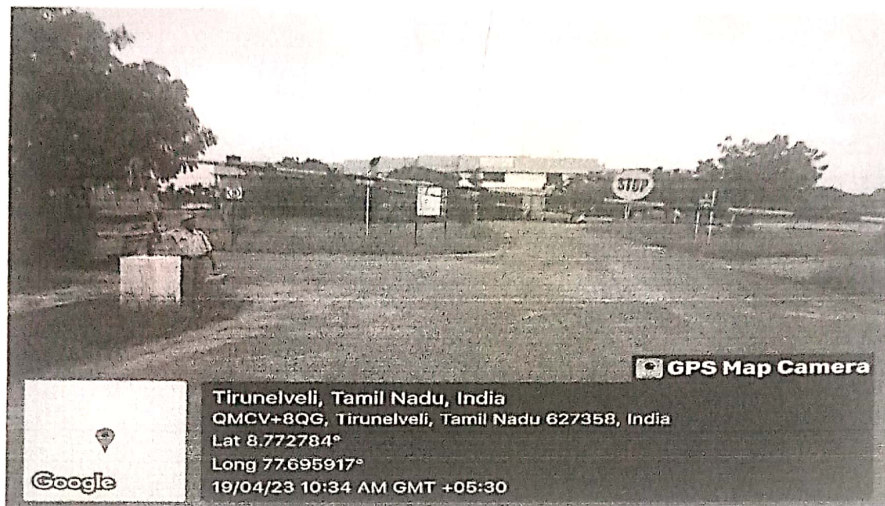
Fig 1: Restricted Entry of Automobiles
