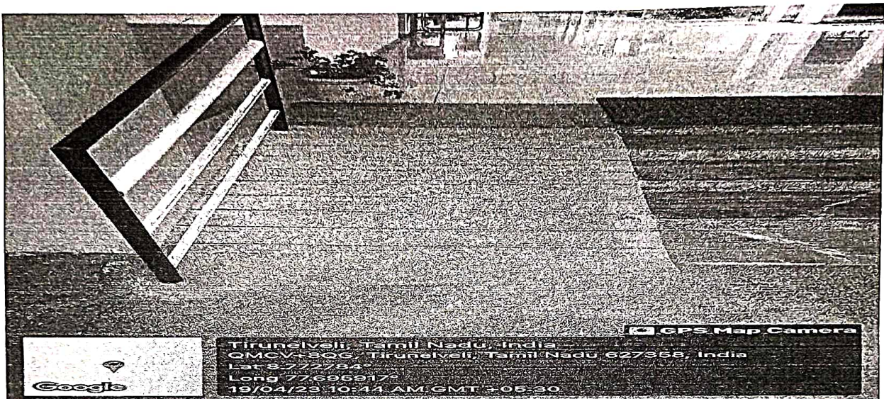
Fig 1.5 Ramp at CSE Block
