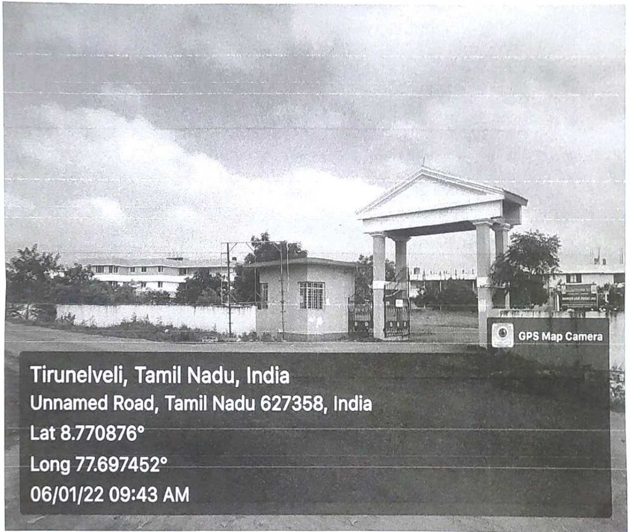
Figure 14. College Compound Wall
