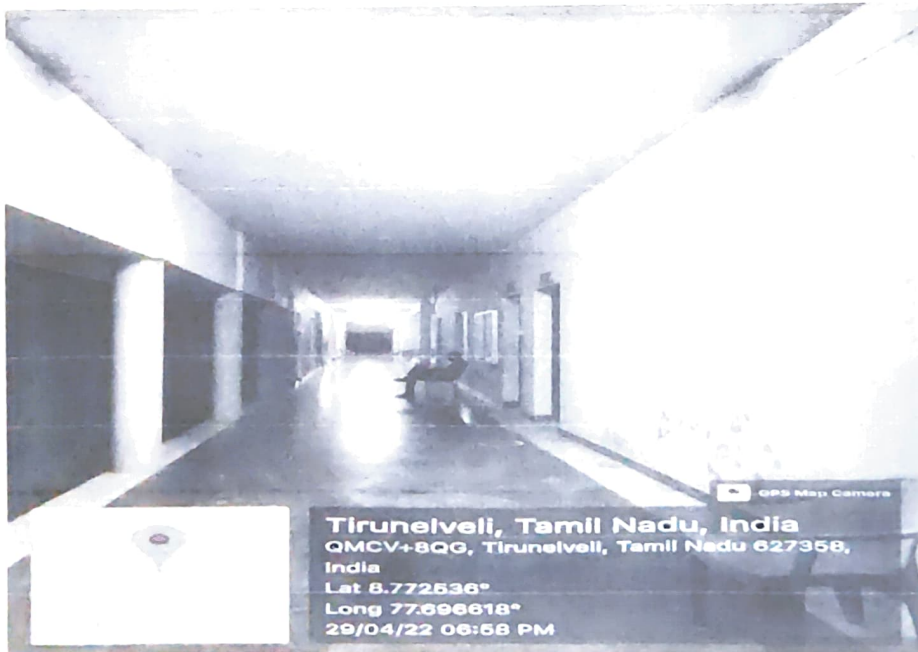
Figure 1. LED in Main Block
