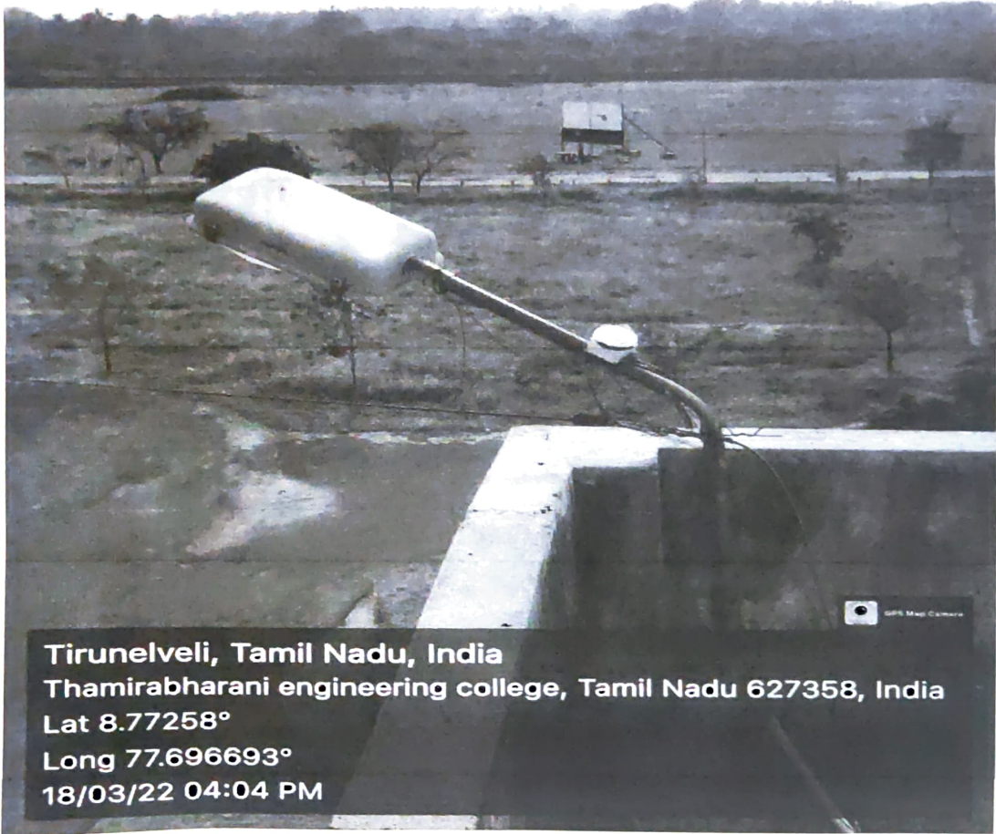
Figure 4: Automatic Street light timer -4 in Main block
