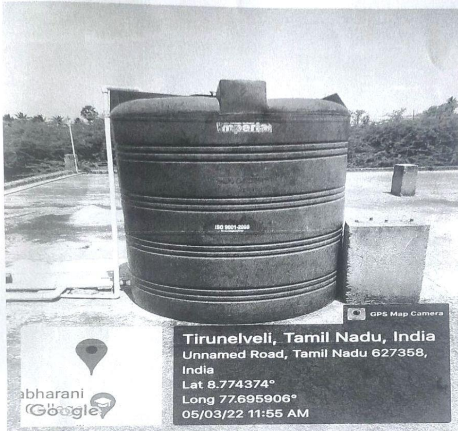
Fig. 7.1.4.21 Water tank in girl's hostel
