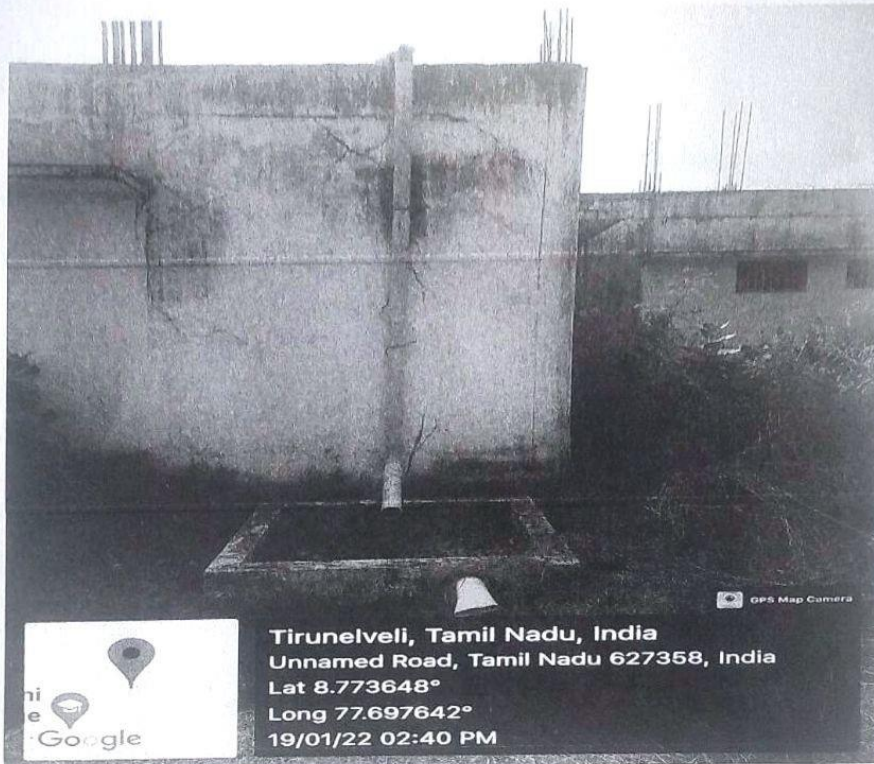
Fig. 7.1.4.5 Rain water harvesting in Boys Hostel
