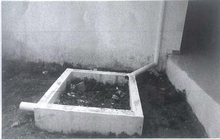
Fig. 7.1.4.1 Rain water harvesting in CSE Block
