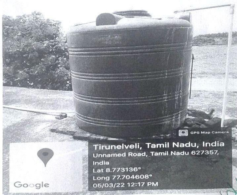
Fig. 7.1.4.26 Water tank in boy's hostel
