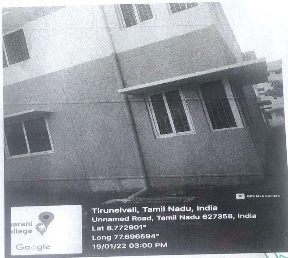
Fig. 7.1.4.4 Rain water harvesting in Main Block
