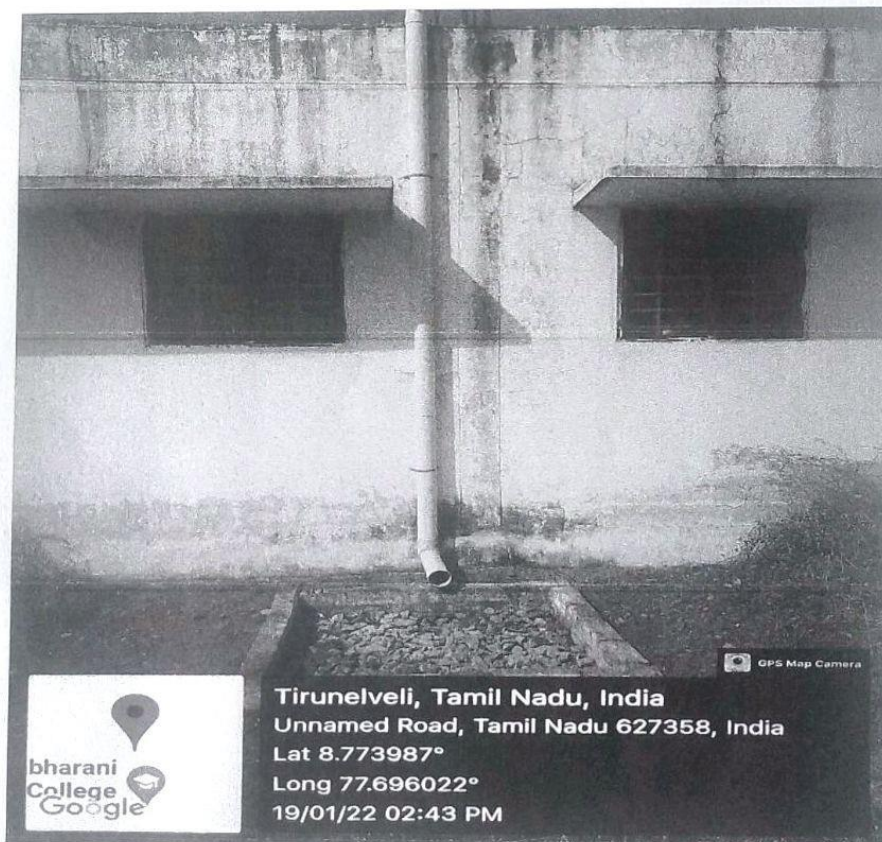
Fig. 7.1.4.6 Rain water harvesting in Girls Hostel
