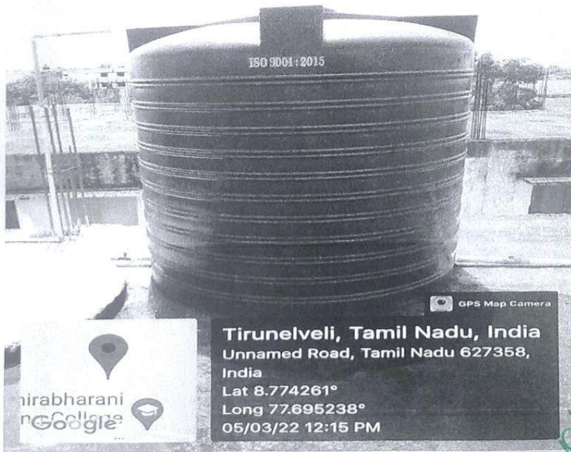
Fig. 7.1.4.24 Water tank in boy's hostel PRINCIPAL THAMIRABHARANI ENGINEERING COLLEGE Chathirampudukulam Village, Chidambaranagar-Vepemkulam Road, Thatchanallur, Tirunelveli - 627 358.
