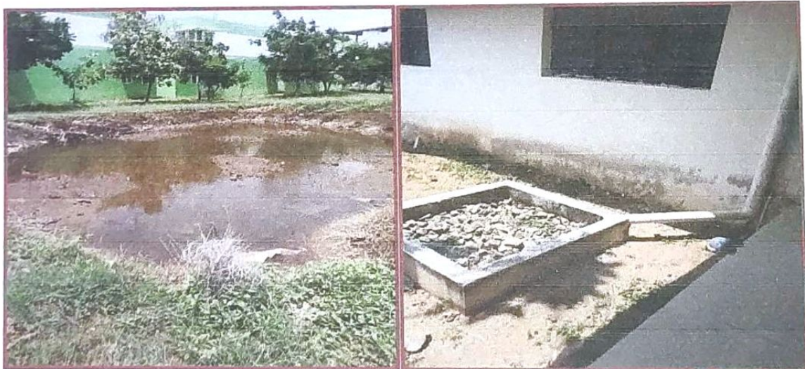
Fig.4: Rain Water Harvesting (RWH) system & Water Body Implemented In the College
